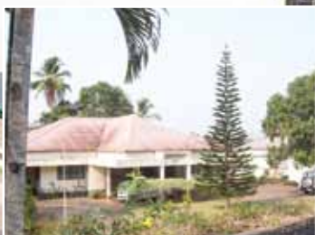
Synthite Calicut plant. (Inset) Administrative block
